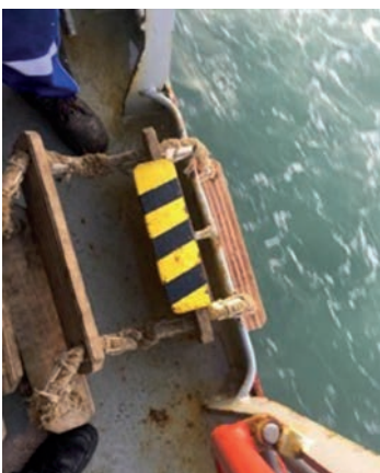
Deck tongue supporting the ladder.
