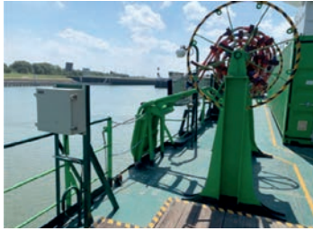
Non-compliant (by design) pilot ladder winch.
